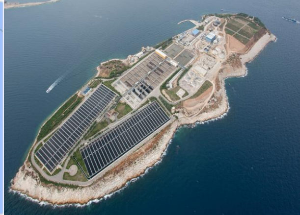
Figure 2: Aerial view of Psytalia Island with wastewater treatment work prior installation of THP
