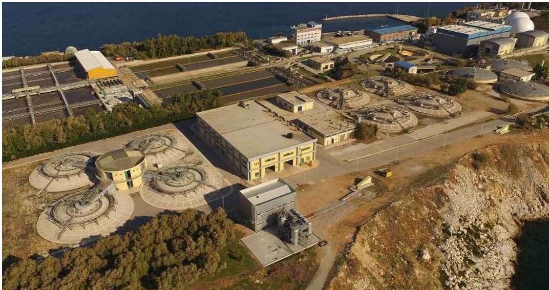
Figure 4: Aerial view of the THP plant (Bottom) and 8 mesophilic anaerobic digesters at Psyttalia WWTP
