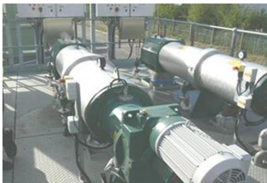
Figure 2 - Sludge Screens
