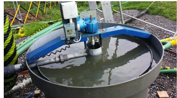
Stage 3b – Radial Clarifier supplied by WRc to overcome excessive sludge build up on Lamella plate clarifier
