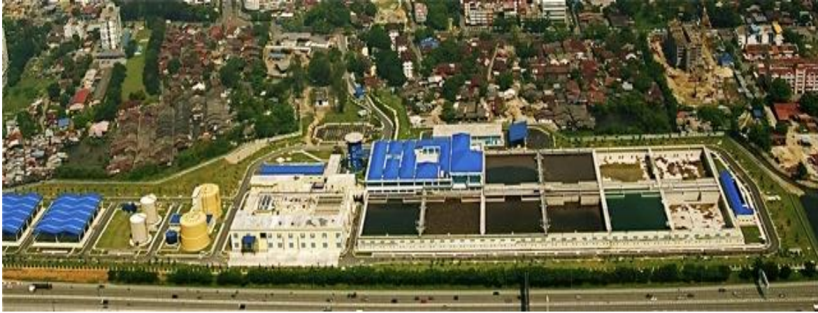
Figure 1: C-Tech configured sequencing batch reactor - Jelutong
