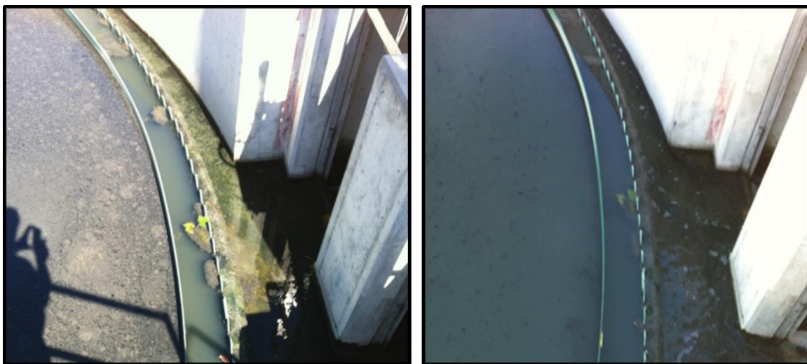
Figure 13. Secondary clarifier before (left) and after (right) introduction of RE technology
