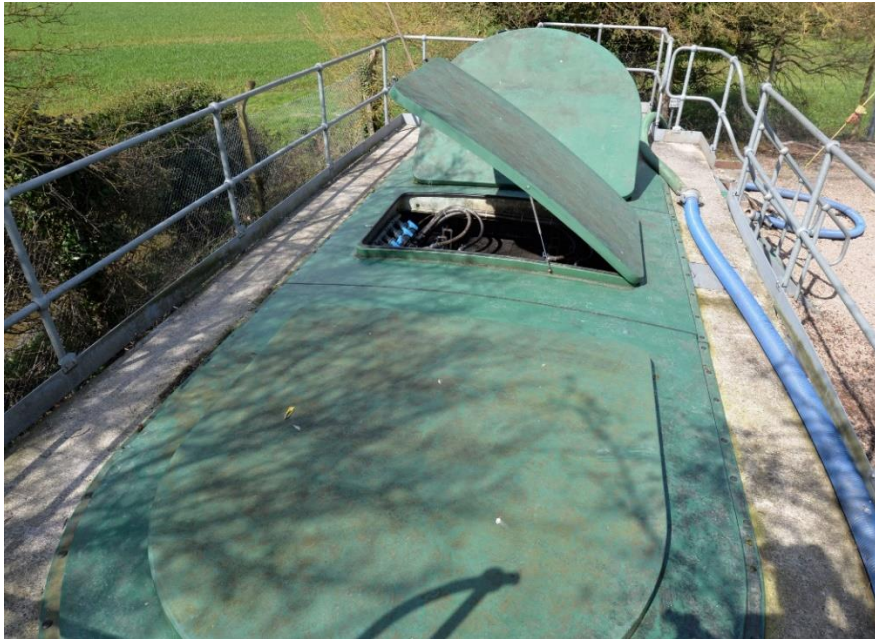
Figure 5: A 15 year old WPL HiPAF® wastewater treatment plant – the refurbishment nearly doubled the flow and load from 100 to 189 PE.
