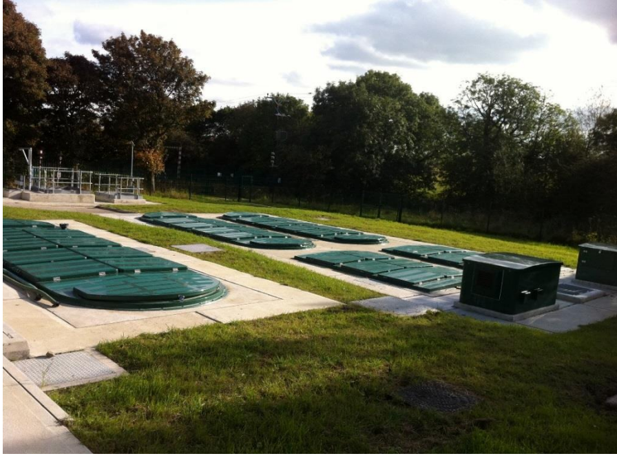
Figure 1: Example of a below ground WPL HiPAF® packaged multi-unit wastewater treatment plant.
