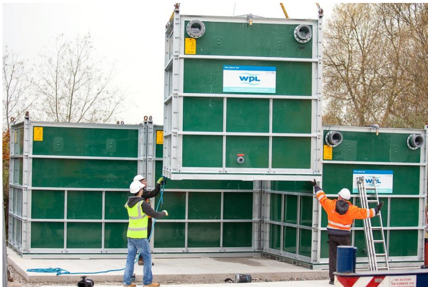
Figure 6: The flexible packaged WPL Hybrid-SAF™ units can be installed in series to form a multi-unit wastewater treatment plant.
