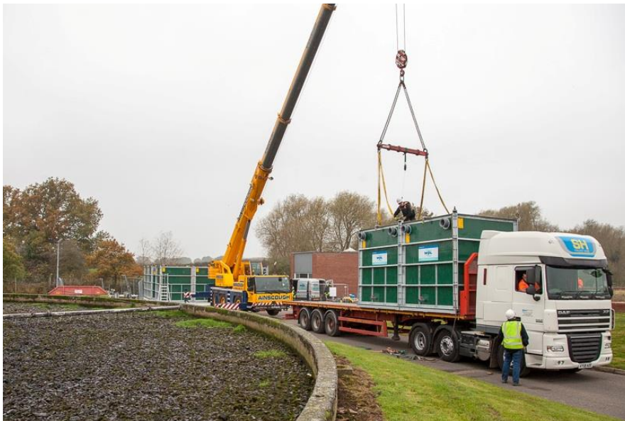
Figure 3: Packaged treatment plants can be easily lifted onsite.
