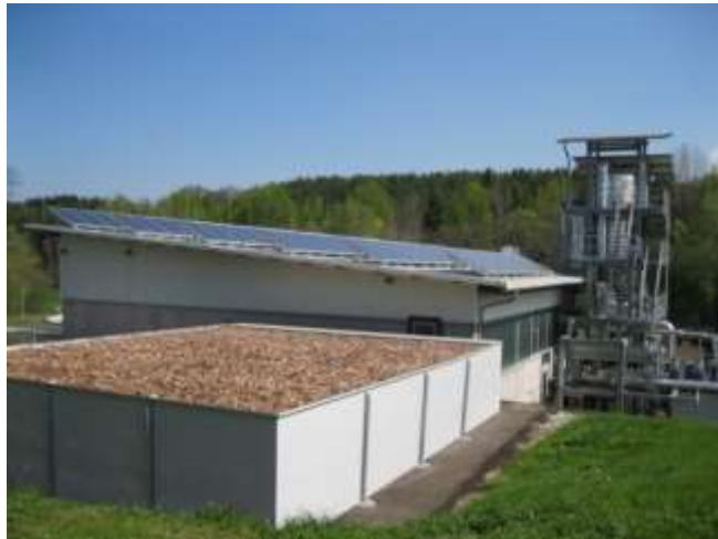
Figure 5: Outdoor bio-filter with wood – chips in open plastic tank
