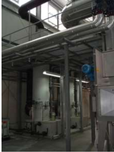
Figure 4: Indoor two stage scrubber
