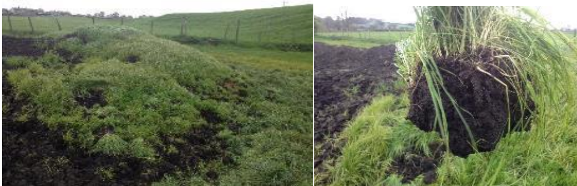
Figure 6: “Live Cover” established on stockpile - Grass roots hold the surface
