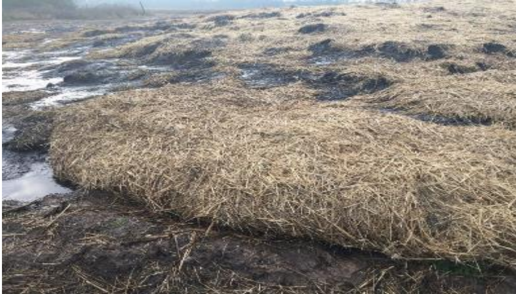
Figure 7: Collapsing stockpile edges forms a fairly strong straw bund
