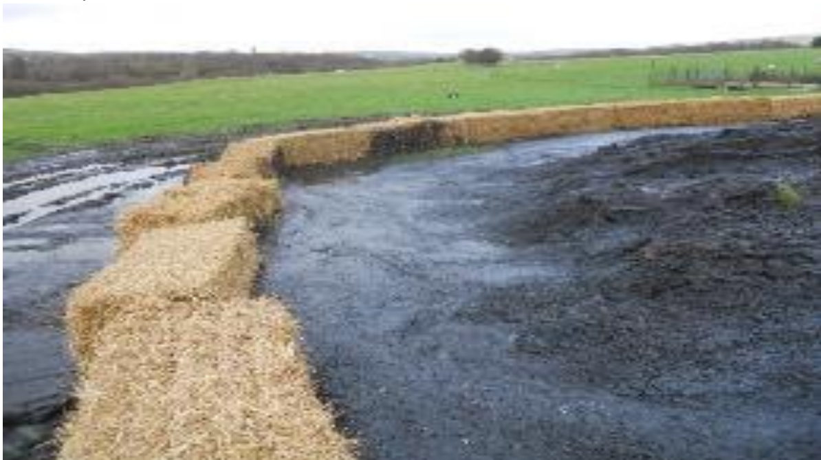
Figure 3: Straw bund constructed around a collapse Biosolids stockpile
