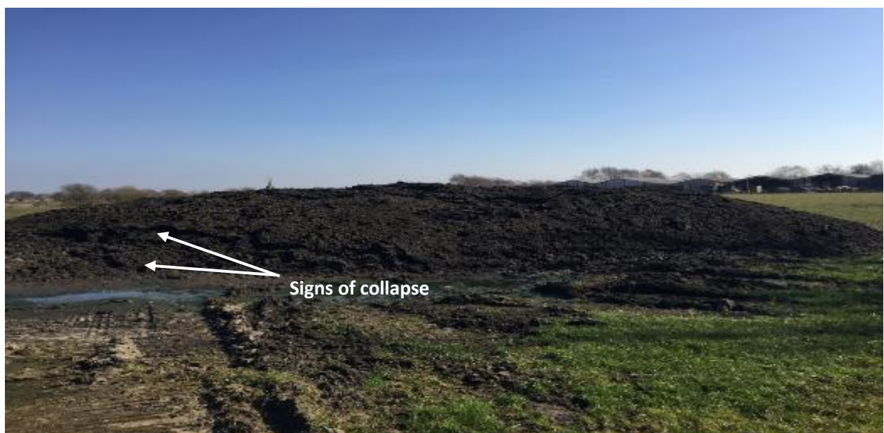
Figure 11: Signs of surface collapse and sloppy area on bare stockpile
