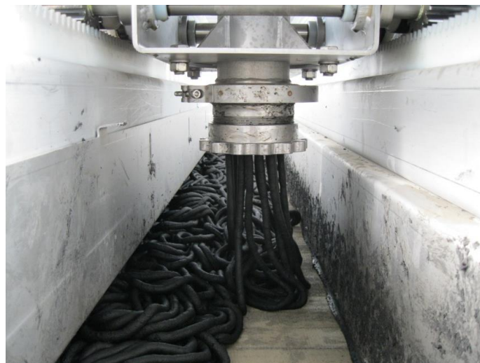
Figure 2: Extruder for dewatered sludge at dryer feeding [HUBER SE 2012-2015]
