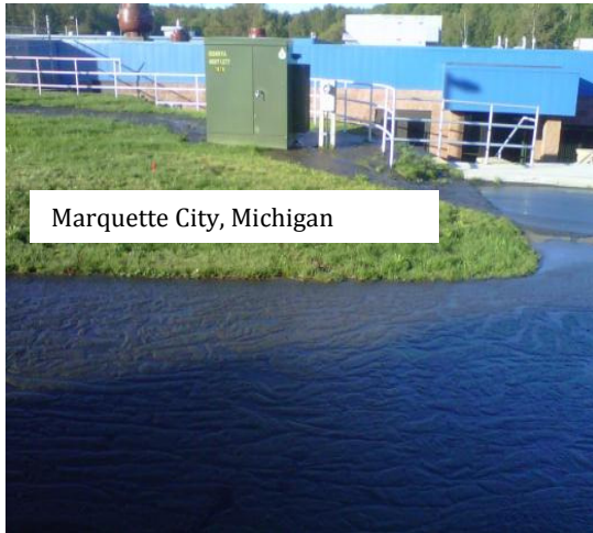
Figure 2: Extreme Impacts of AD Foaming
