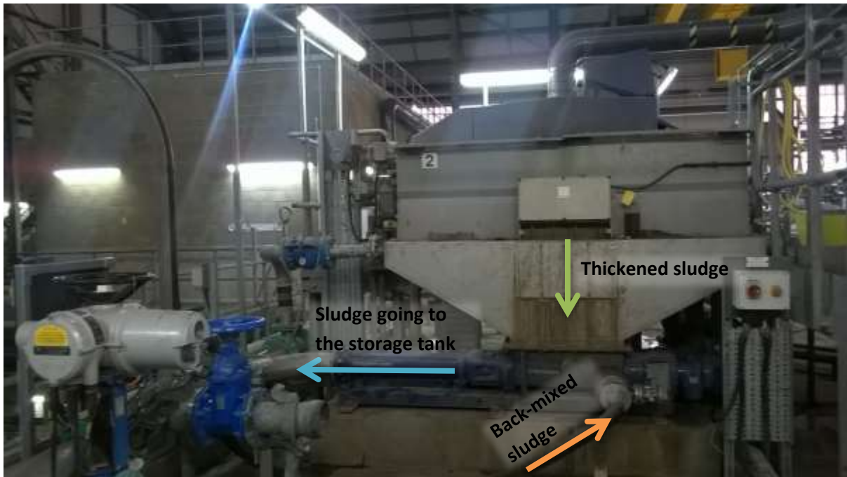
Figure 3: Belt thickener with unthickened PS injection point
