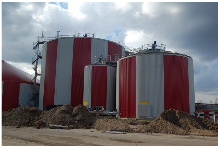
Figure 1: Apeldoorn WWTP, digester tanks
